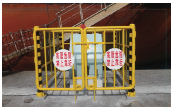
Figure Connecting facilities of the high voltage shore power system.
