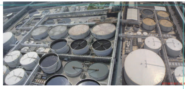
Wastewater treatment plant (Before improvement)
